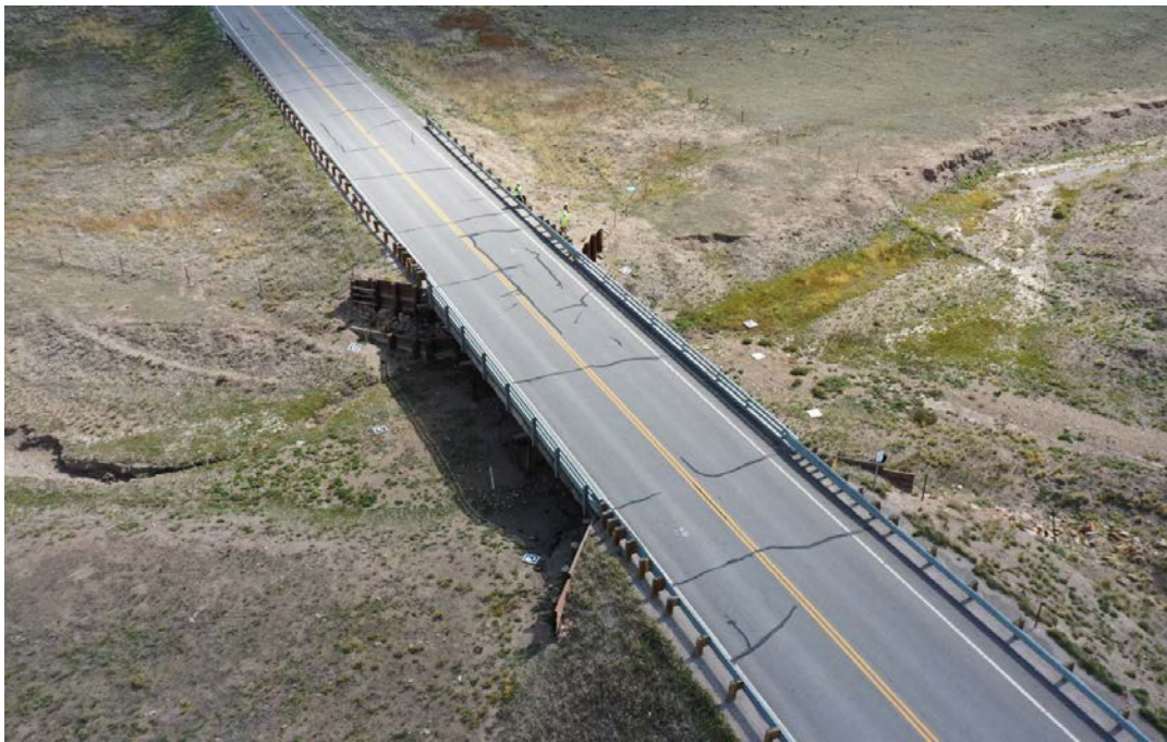
Picture 1 – Bridge I-13-G General Location
