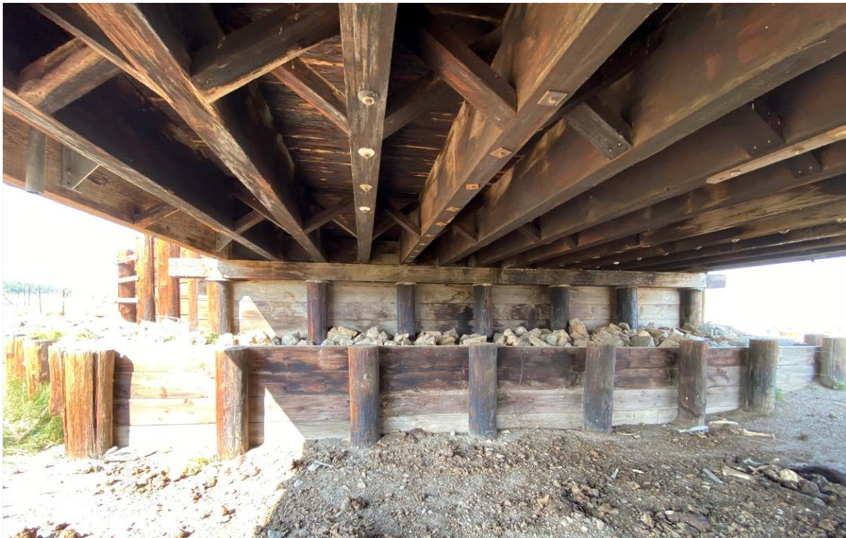
Picture 3 – Existing beam lag bolts
